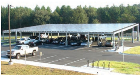
The Marine Corps’ solar roof initiative prompted the addition of this 65-kW solar array on a parking structure at MCAS Beaufort. Photo from U.S. Marine Corps Air Station Beaufort
